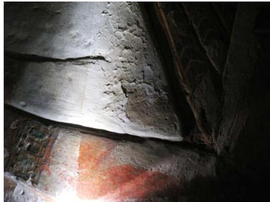
*Detail of a restoration carried out in 1999 showing the addition of white paint and the application of an acrylic consolidant. In raking light it is clear that it is now cracking and peeling from the wall.*
