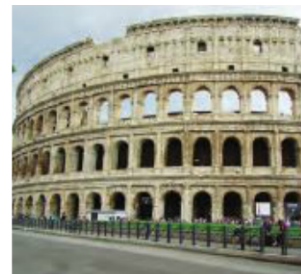
Cleaning the façade is part of the €25m plan
